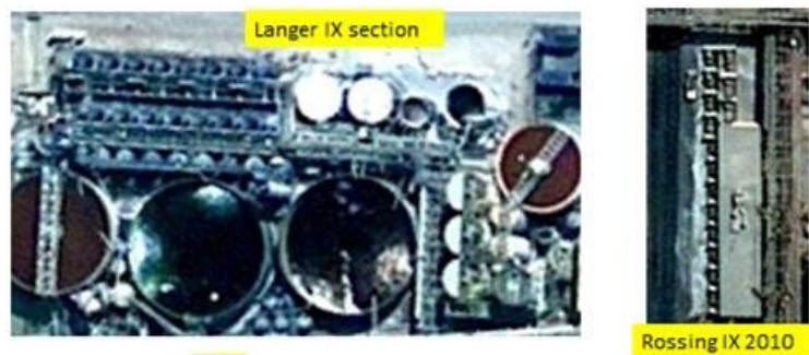
Figure 5 Ion Exchange columns as seen in a GE satellite image
