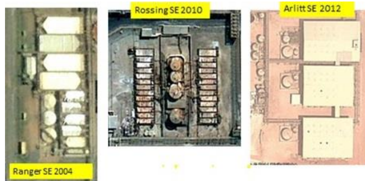
Figure 4 Solvent Extraction Buildings as seen in a GE satellite image
